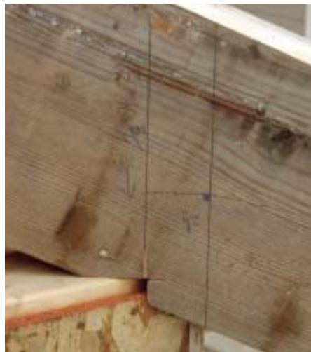
**Figure 6.** Because the heel cut lines have been set back the correct distance on each side, the birds-mouth sits at the exact corner of the wall.
